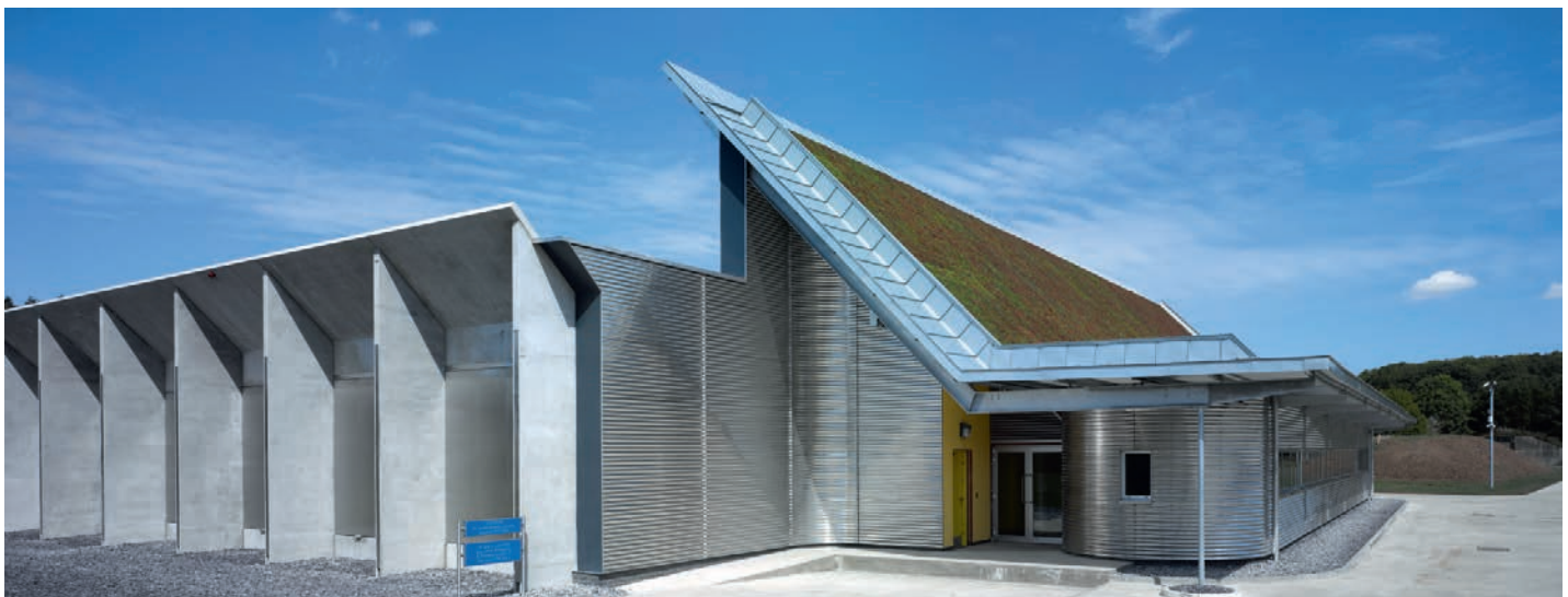
4. Master Film Store: goods entrance at the office end of building with sedum roof and some nitrate pressure relief doors. ©BFI Photograph by Edmund Sumner
