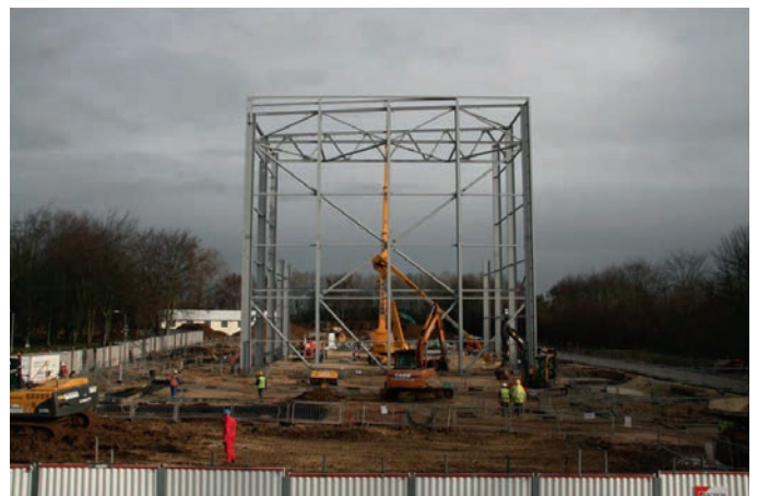
3. The new newspaper storage building takes shape at Boston Spa.
