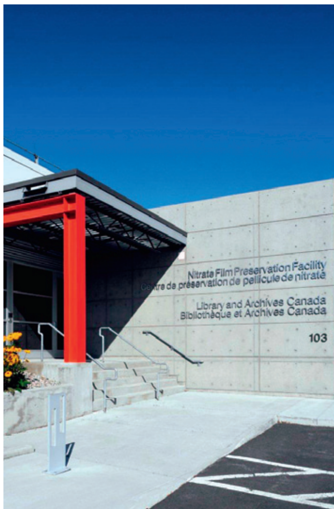
1. Library and Archives Canada's cellulose Nitrate Film Preservation Facility. Photo by Gordon King, 2011.
