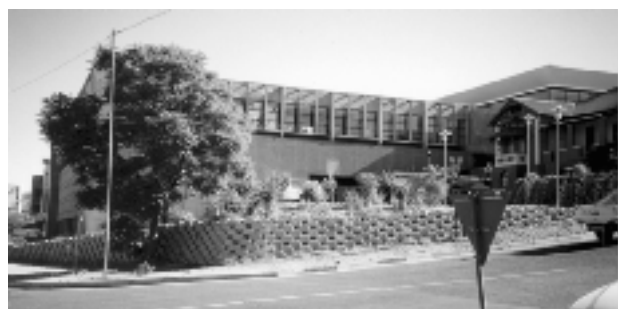
Figure 2. The new National Archives and National Library building in Windhoek, Namibia.
